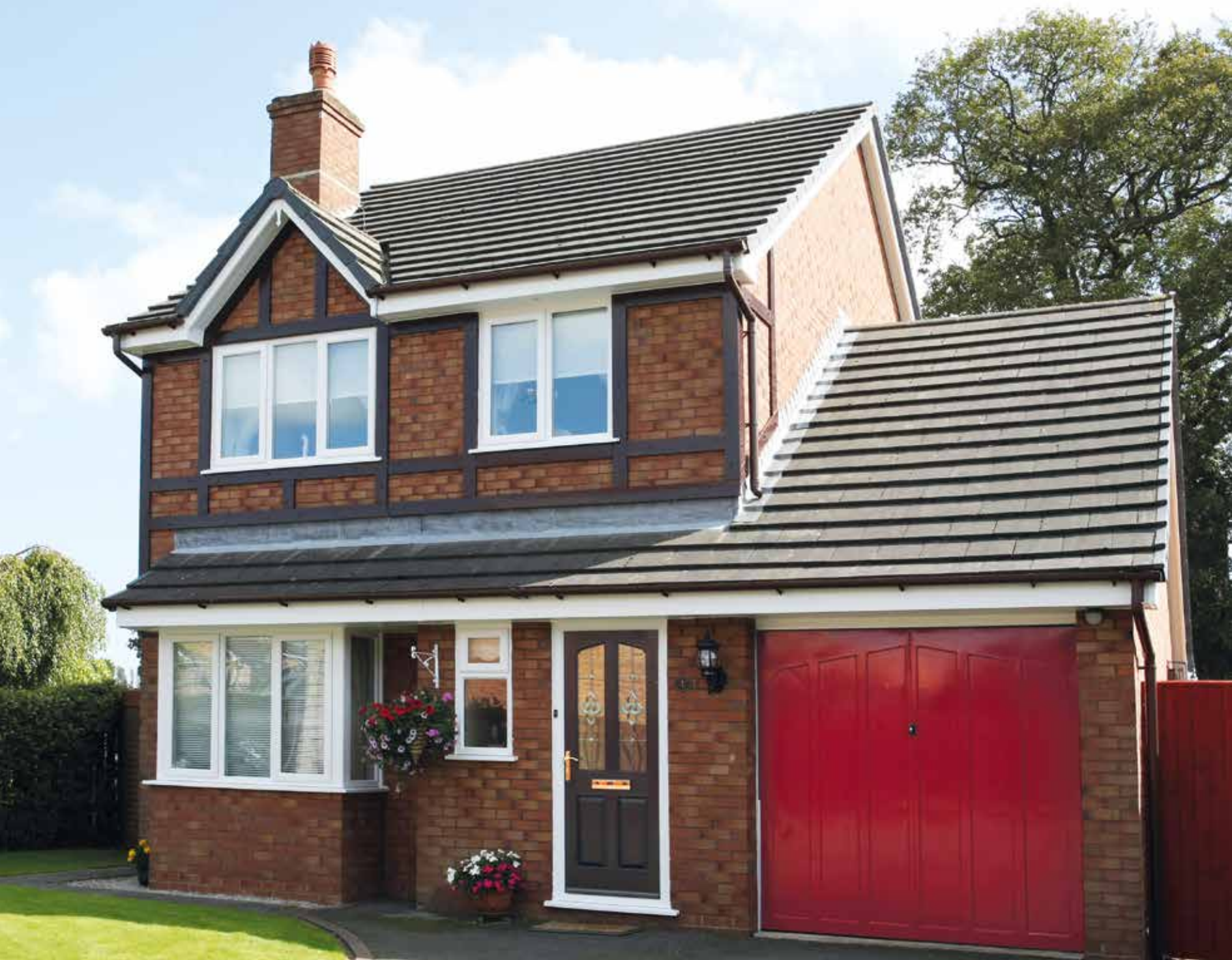
▲ Detached property with White standard fascia boards and hollow soffit boards, finished with half-round guttering in Brown
